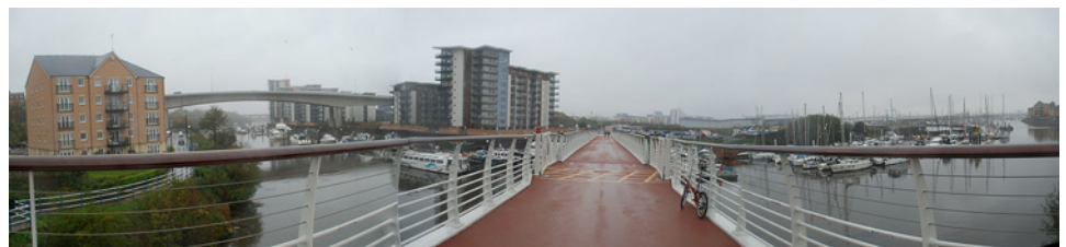
Figure 2 Cardiff case study site. ©Andre Neves. Reproduced with permission.
